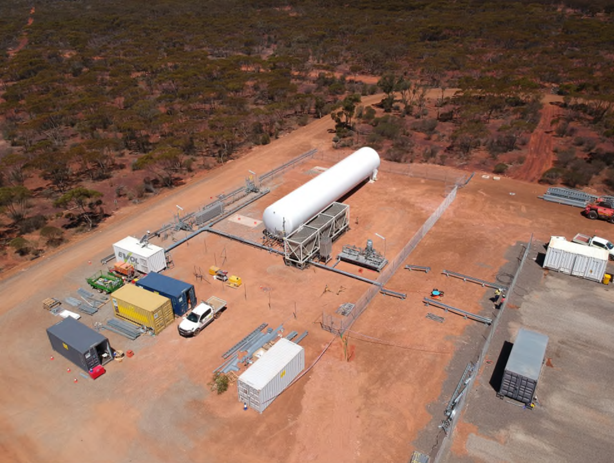
Davyhurst Power Station Construction of LNG Facilities Nearing Completion
