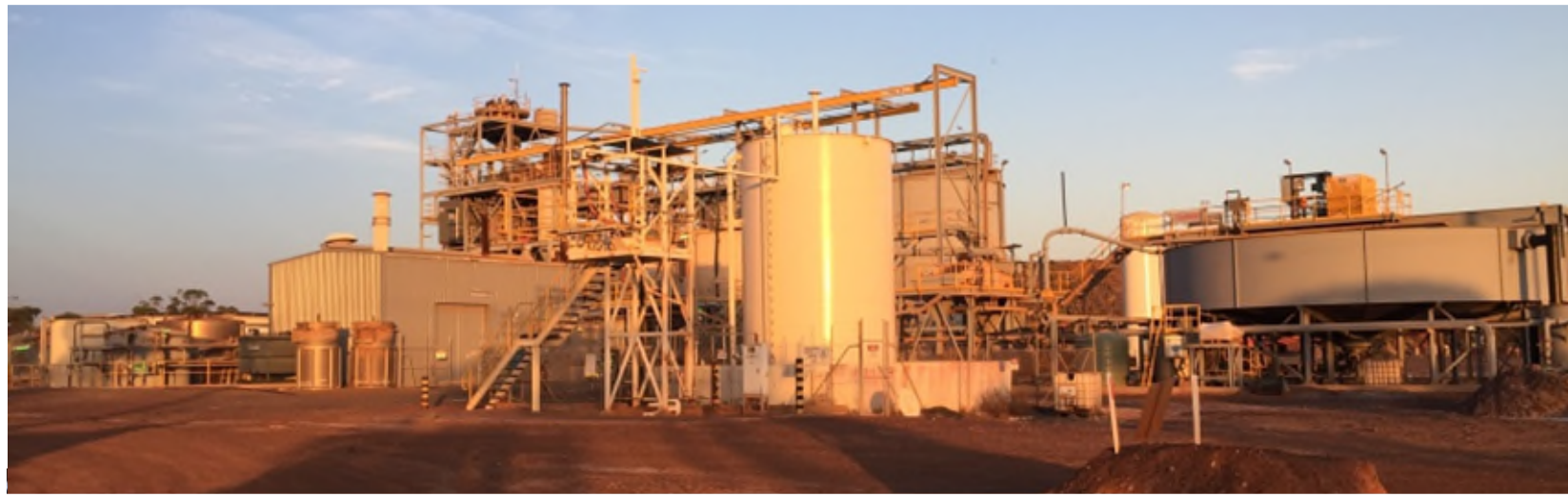
Davyhurst Accommodation Camp
