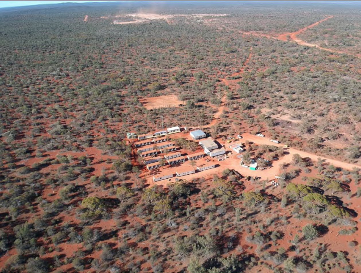
Riverina Camp Establishment of New Camp at Riverina Well Advanced.
